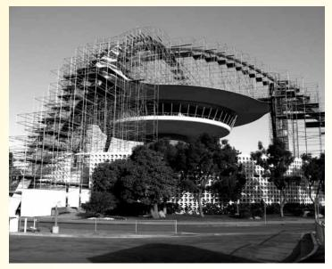
The 1959 Theme Building at Los Angeles International Airport is composed of a reinforced concrete annular core and four steel arches placed at 90-degree orientations.
