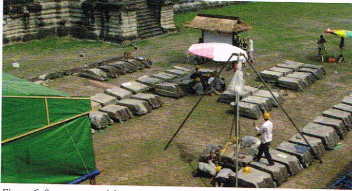
Figure 6: Stones removed from the Angkor Wat roof structure being conserved in the on-site workshop. Courtesy of the World Monuments Fund.
