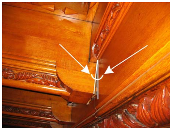
Figure 1. Open joint in the decorative trim of the lower chord of truss #3.
