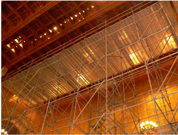
Figure 3. Scaffolding positioned below the ceiling truss
