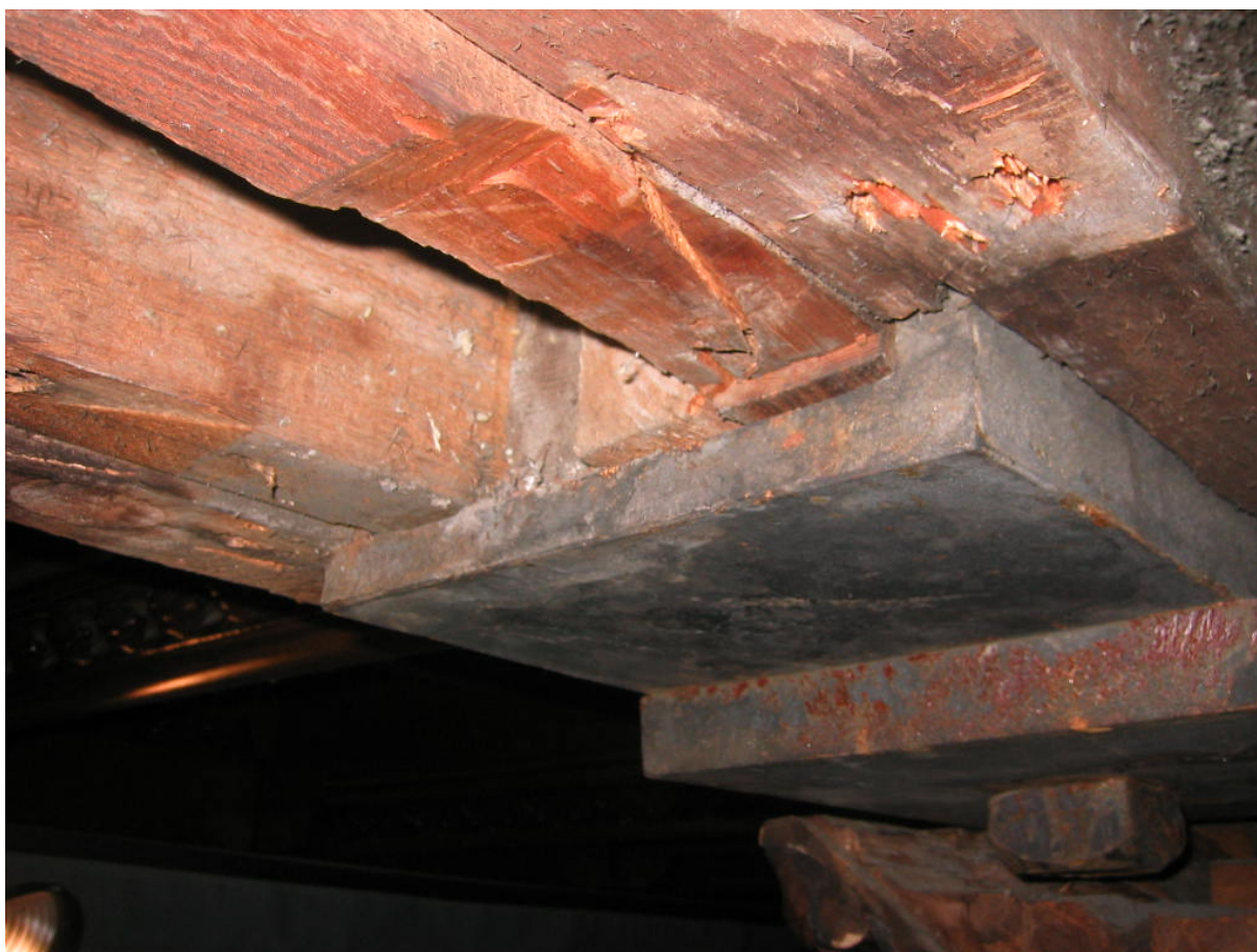
Figure 11. Split bottom chord, east end of failure
