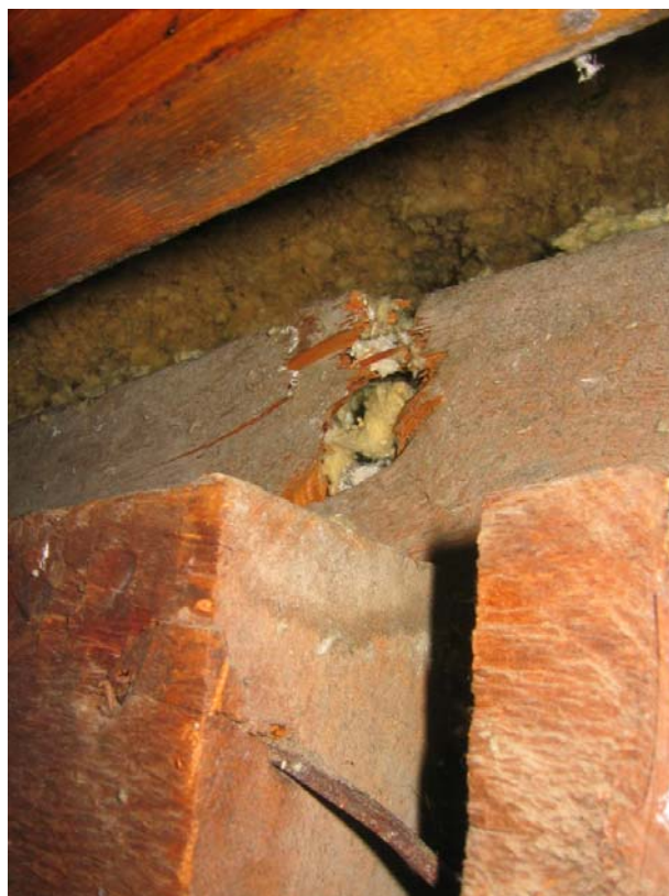
Figure 12. Split bottom chord, west end of failure
