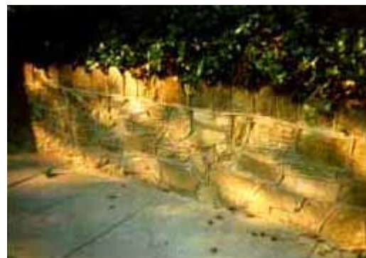
When repairing this stone wall, the mason matched the raised profile of the original tuckpointing. Photo: NPS files.
