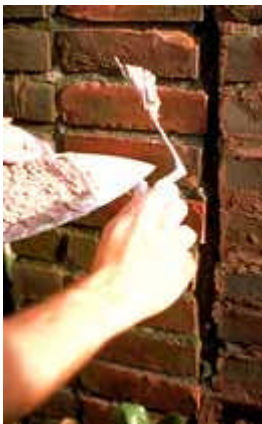
This mortar is the proper consistency for repointing historic brick. Photo: John P. Speweik.
