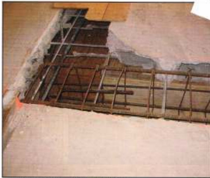
Strengthening of existing slab (Slag Block System).
