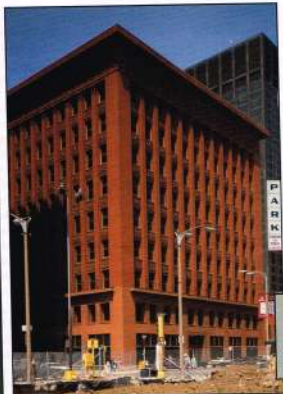
20 th Century Loadbearing Masonry Building
